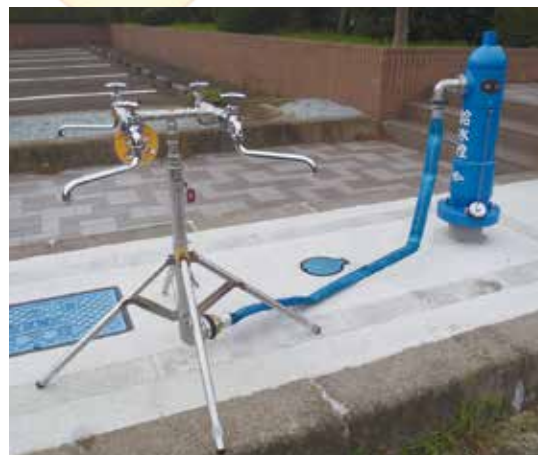
災害時給水栓 Disaster Water Taps
